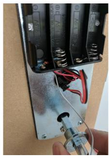
6. Fit the interior fixing plate and alignment insert over the spindle. Screw in the 3 fixing bolts, make sure these have been cut to the right length. See installation instructions. Connect the power cable and the remove the alignment insert.
