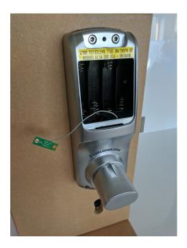
7. Fit the internal lock body, carefully pull through the wifi cable. Tighten the 4 allen screw bolts.
