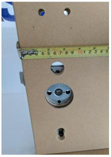
1. Fit the Salto latch as per the enclosed instructions. It is backset 60mm. Offer up the paper drillling template that is included with the 7i and drill as above.
