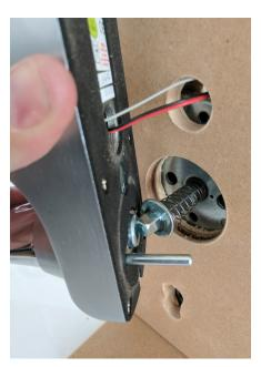
4. Thread the power cable and wifi antenna cable through the top hole. Insert the spindle into the spindle hole on the keypad and offer up to the door.
